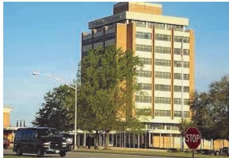
US Army 11 Building Renovation Project Ft Gordon
