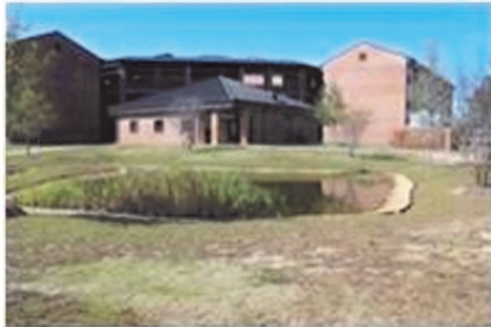
120 Person Dormitory, Moody Air Force Base
